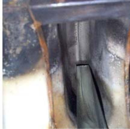
The flame deviation test is the second listed AGA inspection step. Should the burner flame move when the circulator blower comes on it is an indication of a heat exchanger leak. If you do not locate a crack or perforation the heat exchanger seams may be leaking and the cause for the flame deviation, or the metal may have pinholes rusted through the wall.
